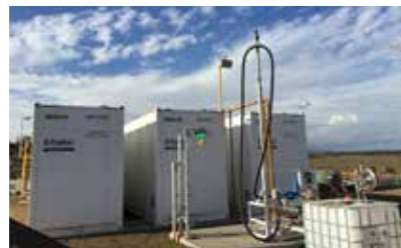
Mine Site Refuelling Facility Australia
