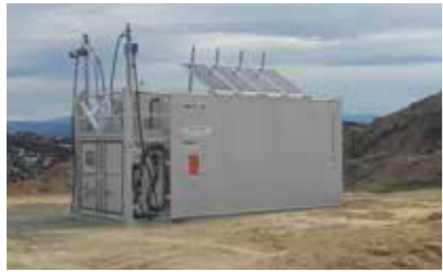
Solar Tank for Farming Client New Zealand
