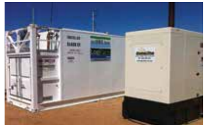
Back-up for Power Generation Australia
