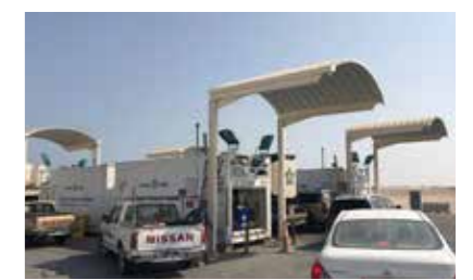
Modular Service Station Qatar
