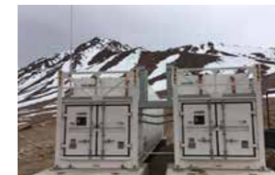
Remote Fuel Station for Mine Chile
