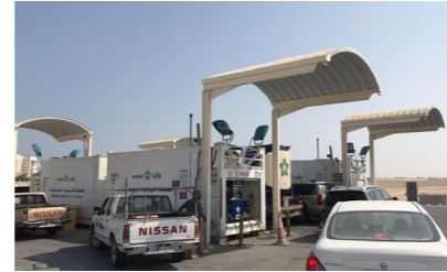
Modular Service Station Qatar
