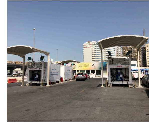
MODULAR FUEL STATION, QATAR
